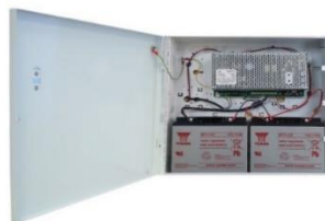
Figure 7 – Battery backup supply
